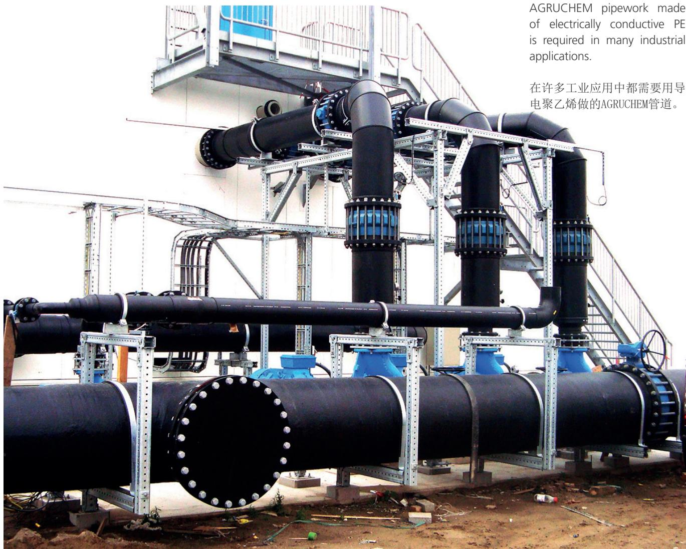
AGRUCHEM pipework made of electrically conductive PE is required in many industrial applications.
