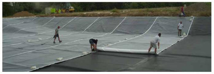
HDPE geomembranes act as a seal for central ground filters that collect rain water from flight operation areas with contamination from surface de-icing.
