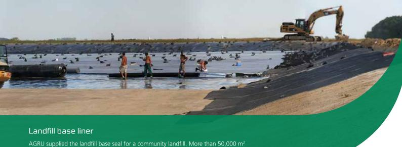
of 2.00 mm HDPE geomembranes, both smooth and textured, were installed here.
