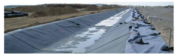
Local ground filters are also being made from HDPE geomembranes to go next to the runways and taxiways. These are being used to treat rainwater with impurities from flight operations and surface de-icing before it is transferred to the central ground filters.
